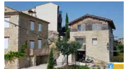
La Tour, Faucon, Mistral Habitat F. Chabert, C. Mendez, architectes
